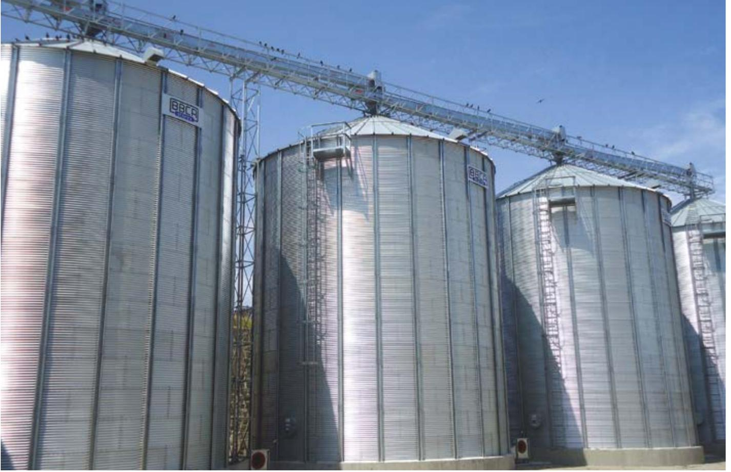
Flat Bottom Silos deliver diversity by involving easy assembly resulting in minimal installation costs and highly efficient low cost storage.
