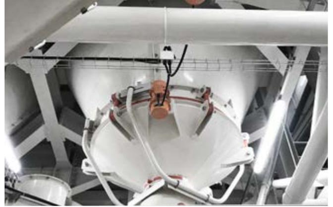
It is used in depots on a free circulation, in a way to discharge the product (flour, wheat, bran, etc.) very easily. The outlet which is connected with joints to the body is vibrated by a Vibro motor. Thanks to this vibration, the products in the store flow down and gets easily discharged into the screw or conveyor.
