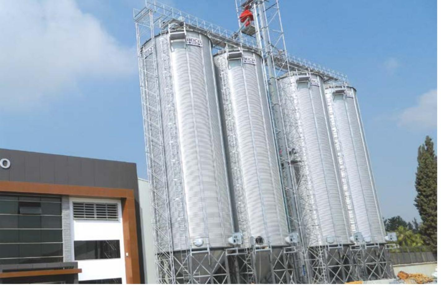
Hopper Silos are typically used in applications where routine and fast clean out is required or just to reduce the energy and labor cost of material handling.
