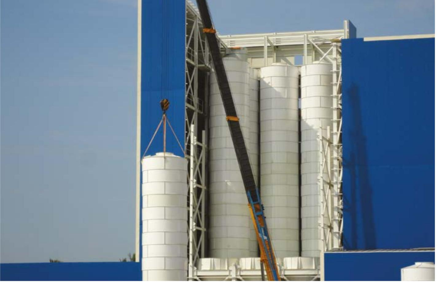
UĞUR offers solutions to its customers with steel silos in order to store flour, bran, semolina etc. granular and powder products. It is manufactured in modules with all bolted combining. Mounting and demounting can be made easily. Modular system is adapted according to customer request. It is designed in demanded sizes and requested capacities.
